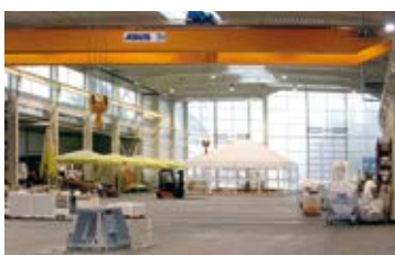
2x25 t Hallenkräne 2x25 to overhead cranes
