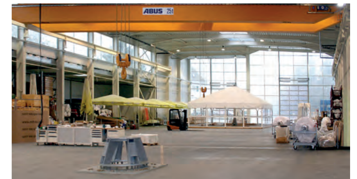
2x25 to overhead cranes
